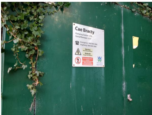
Figure 16: Pumping station at Cae Bracty
